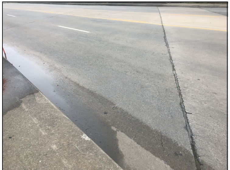
Span 1, transverse deck cracks.
