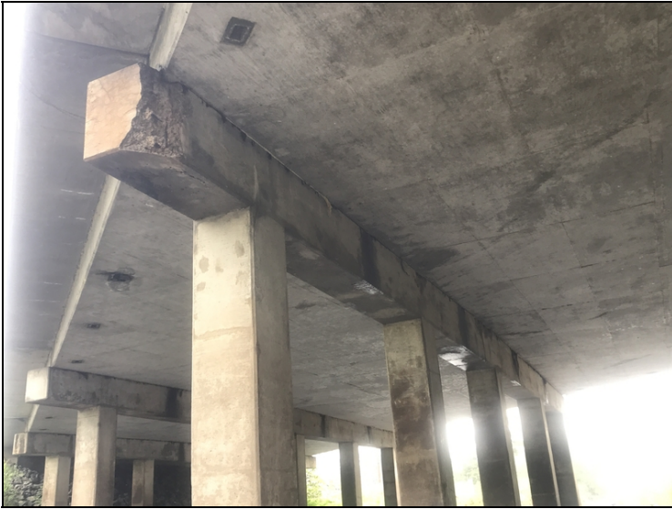
Bt. 3 cap, back side has spalls with exposed rebar.
