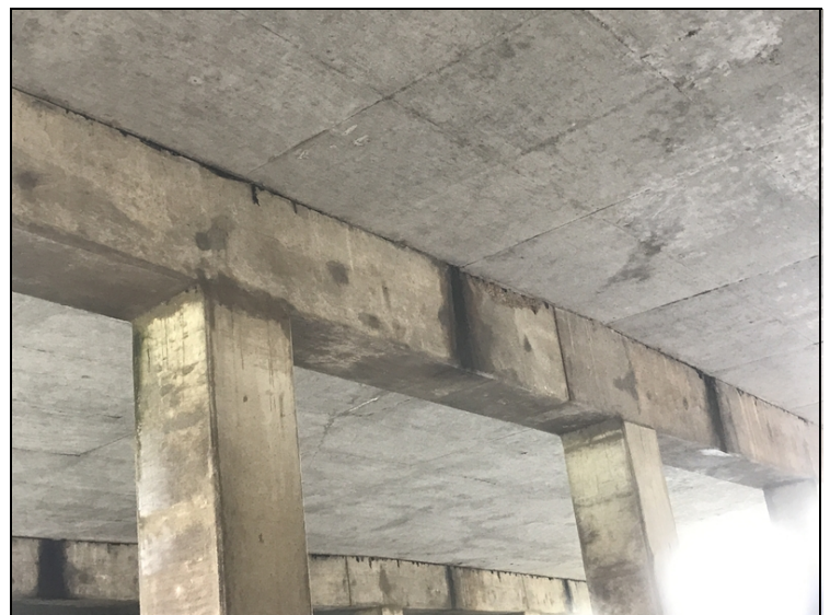
Bt. 4 cap, back side has a spall.
